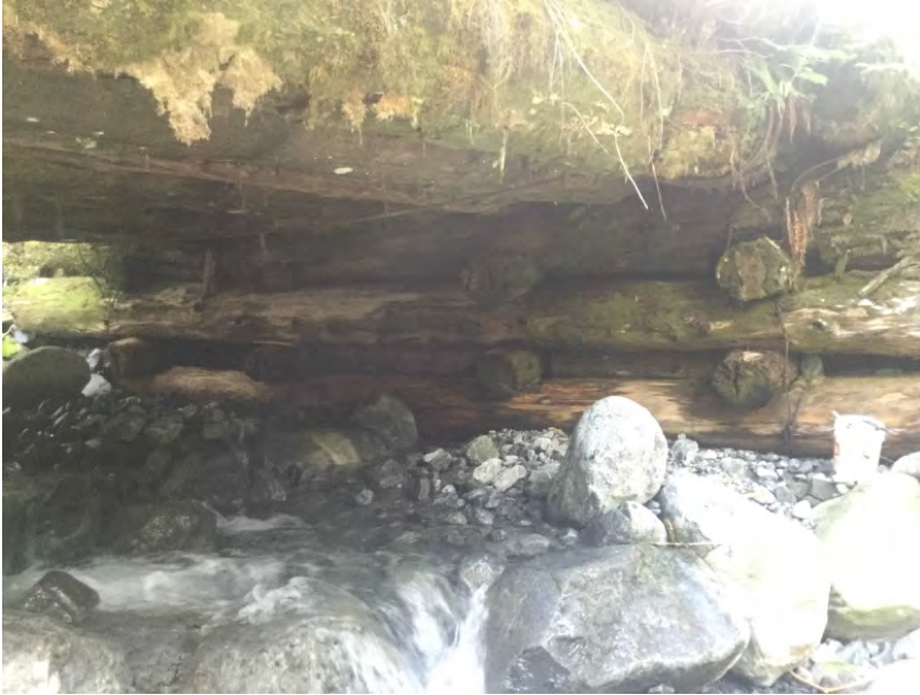
Left Bank Abutment
