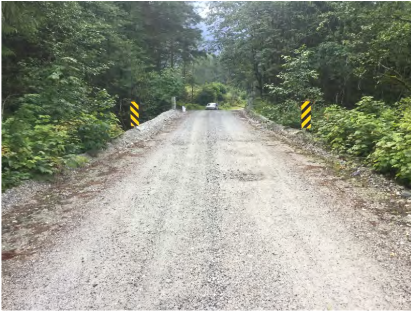
Right Approach Facing Bridge
