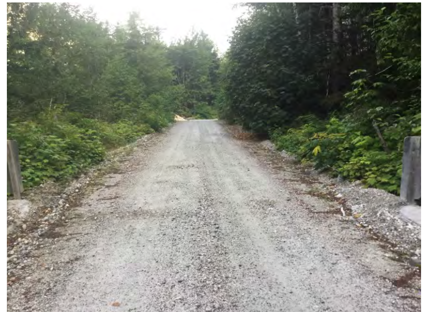
Right Approach Facing Away From Bridge
