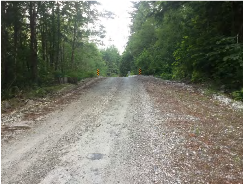
Left Approach Facing Bridge
