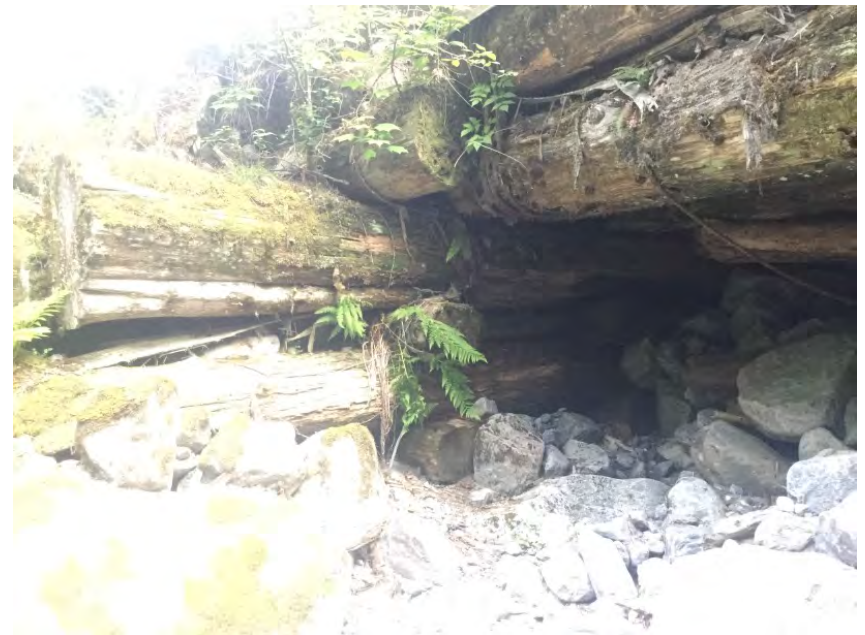
Right Bank Abutment
