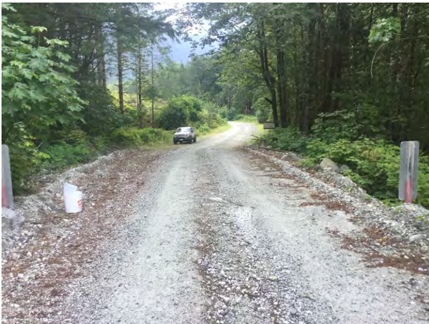
Left Approach Facing Away From Bridge
